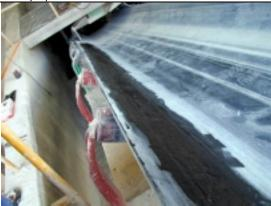
Eli-Flex has the viscosity of toothpaste so it is easy to work on slopes, vertically and even upside down. Eli-Flex only requires 2 hours for every 2mm or  $1/16^{th}$  of depth of the repair. Eli-Flex cures to a Shore hardness of 60-65 depending on the ambient temperature. This superior elongation of 190% mean that Eli-Flex will not "pop out" when the belt wraps around the pulley
