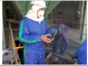
The easy to use packaging of the Eli-Flex product allowed for the exact amount of product to be prepared for each stage. The exact ratio of Epoxy to hardener is in the bag ready for mixing. There was no wastage due to product curing while the belt was being staged, cleaned and prepared
