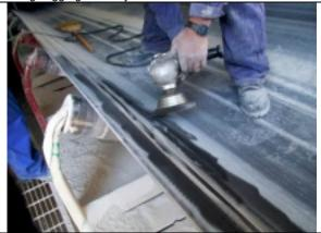
A wire brush attachment was used on an industrial grinding machine that was set to the lowest possible speed. Care was taken not to melt the rubber or further damage the fabric of the belt. There was a lot of dust present so a solvent was used to clean off the area before the Eli-Flex was applied.
