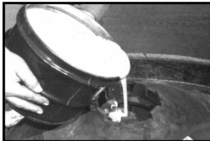
**6** Pour immediately after mixing. Working life is 10-15 minutes after mixing.
