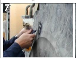
Cut open a corner of the bag and apply a liberal amount to the center of the gouge. You have 20-30 minutes of working time.
