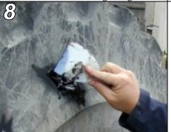
Use your spatula to force the Eli-Flex into the gaps by working from the center outwards. This will help reduce air entrapment and bubbles forming.
